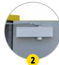
2 Self-closing door with thermo-fuse
